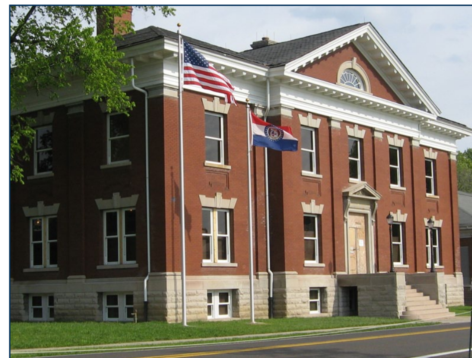
Above: The 1905 Post Exchange and Gymnasium Building at Jefferson Barracks before restoration.
